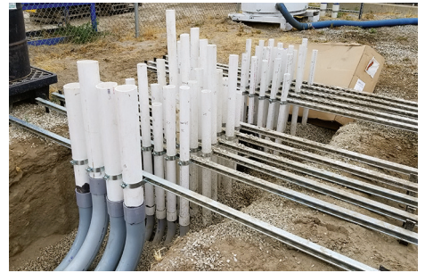
Installation of Remediation Wells
