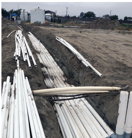
Installation of Remediation Piping
